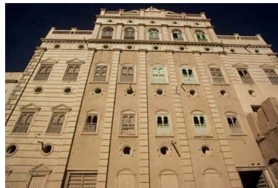
Fig. 4: Dar bin Sahil is an impressive abandoned mansion in fair condition.
