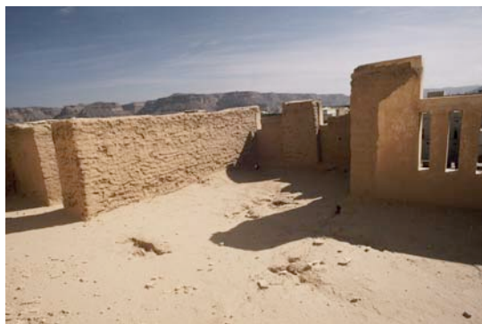
Fig. 35: The roofs of al-Riyad are in dangerous condition as exhibited by these sink holes.
