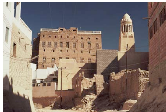
Fig. 16: The area around the Sarjis Mosque is part of the historic core of Tarim, but is in fair-to-poor condition.
