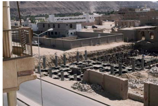
Fig. 20: New unsympathetic concrete construction has compromised the context of Dar al-Salam mansion.
