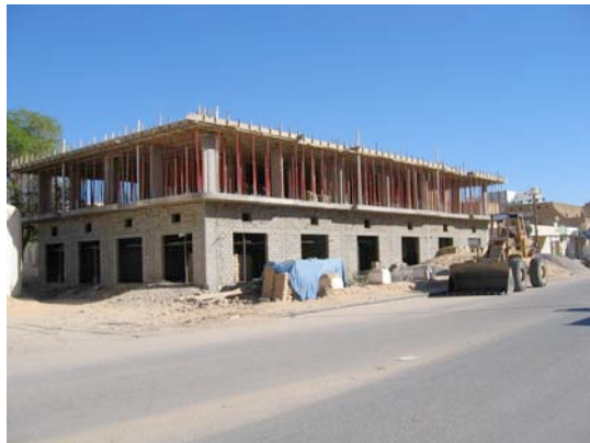
Fig. 19: Unregulated concrete construction across from al-Tawahi in a former palm grove.
