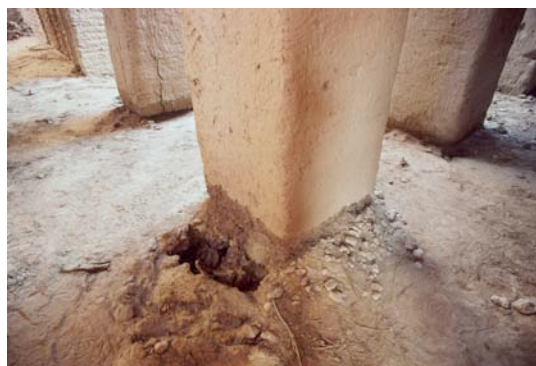
Fig. 30: The massive piers supporting the Hamtut's northwest kitchen wing are severely undermined, risking further collapse.
