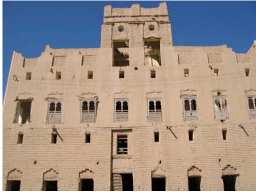
Fig. 13: Bir Yimani is an al-Kaf mansion located in the palm groves on the outskirts of Tarim. The 2000 feasibility study assessed it as beyond repair.
