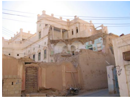
Fig. 18: A portion of the northeast wing of al-Ranad palace has collapsed.
