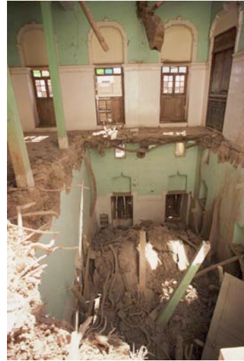
Fig. 2: An area of al-Fijr collapsed as a result of a termite-infested beam.
