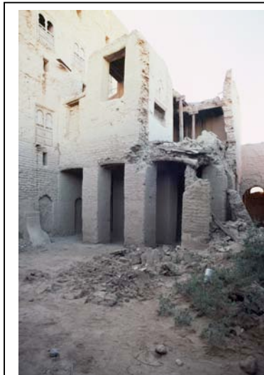
Fig. 29: The northwest kitchen wing of the Hamtut collapsed in 2003.
