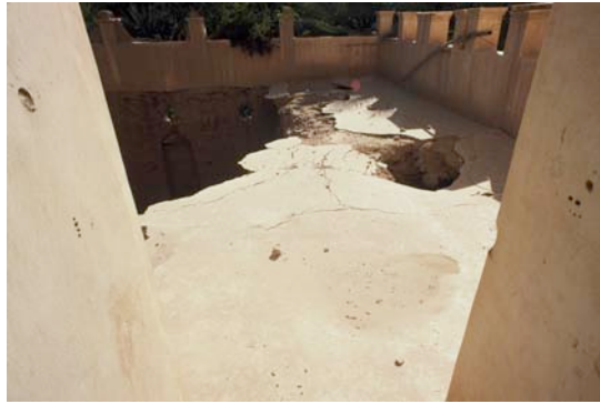
Fig. 5: Some of Dar bin Sahil's terraces are in extremely poor condition.
