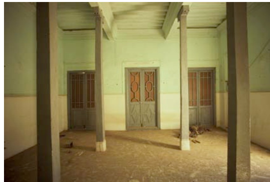
Fig. 28: The Hamtut's 1 st floor west reception room leads to a large terrace with a separate ground floor entrance for the women. Both reception rooms have been remodeled with Art Deco doors.
