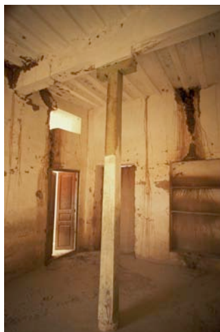
Fig. 36: The interiors of al-Riyad exhibit extensive damage as a result of leaking roofs.
