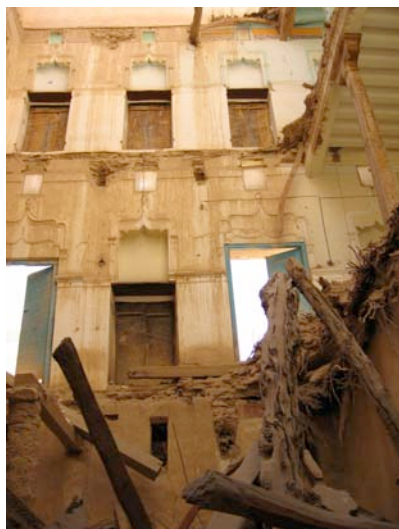
Fig. 9: The northeast area of Dar Mihdhar has collapsed.
