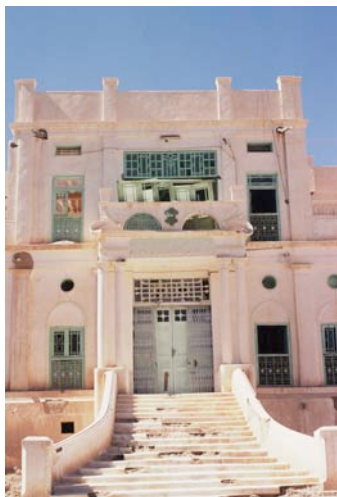
Fig. 15: Al-Haddad, an Art Deco mansion, has suffered the collapse of its balcony doors.
