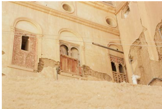
Fig. 7: Lime plaster window inserts are an interesting detail of Dar bin Sahil.
