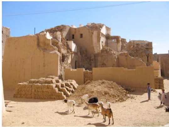
Fig. 17: In the historic core of Tarim, near al-Ranad palace, there are many abandoned and collapsing traditional buildings.
