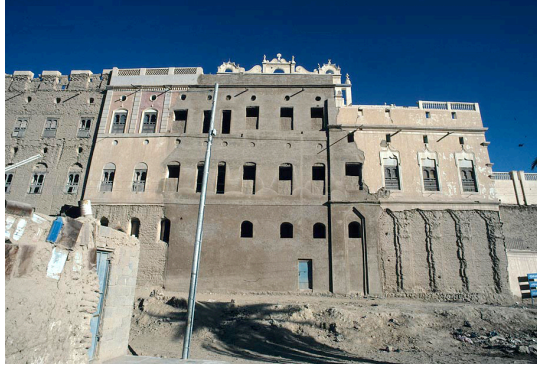
Fig. 1: The collapsed area of the west elevation of the 'Ishshah was reconstructed in 2003 under the supervision of master mason Karami Faraj al-Tamur with funds from the Social Fund for Development.
