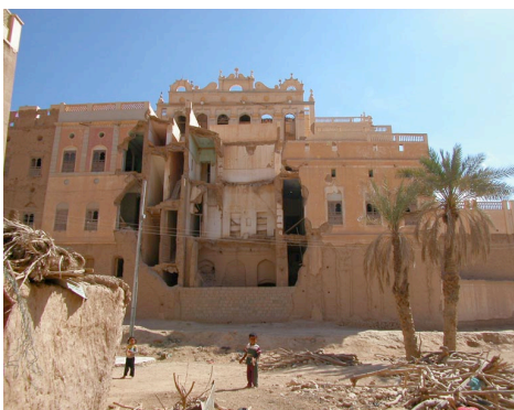
Fig. 9 Collapse, western façade.
