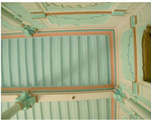
Fig. 7 Lime plaster decoration on interior ceiling.
